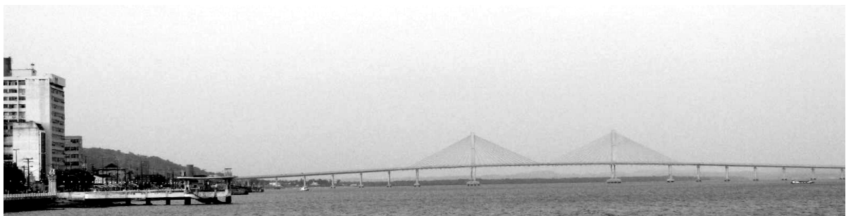
Fig. 4 The Emperor Bridge (first layer, left side) and the Constructor Bridge (back layer). Source: by the authors (Photo: M.C. Giacomet, 2009).
